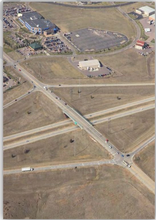
I-229 Exit 9 (Benson Road) Interchange
